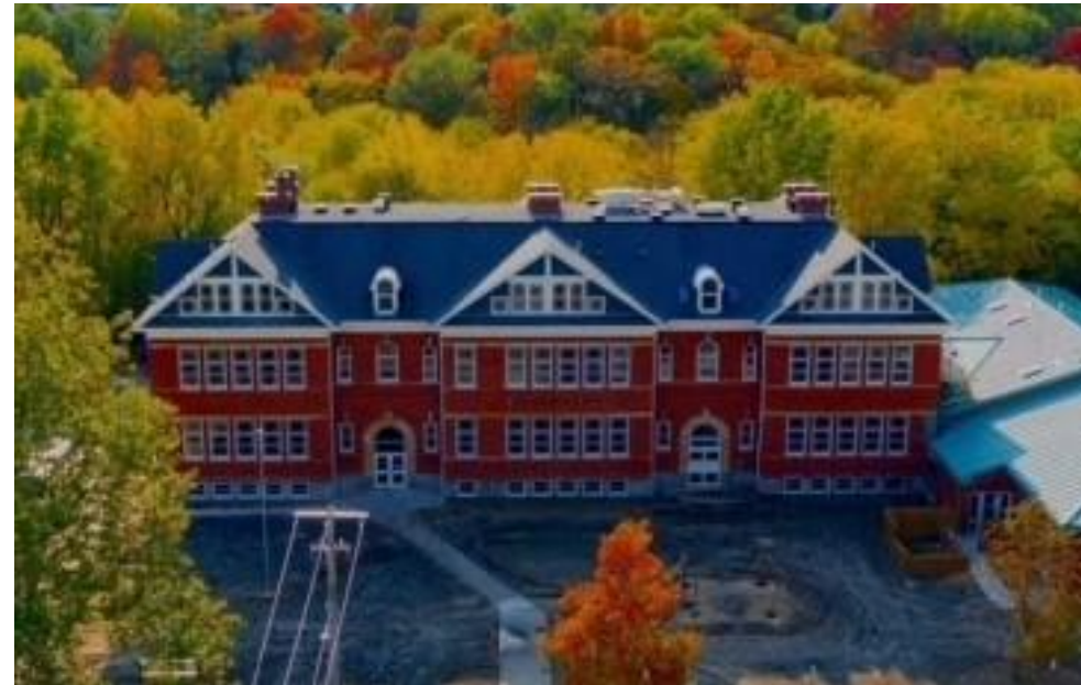
Oxford Estates Integrating Tillsonburg's Rolph Street Public School into new residential apartments - Winner of the Paul Oberman Award for Adaptive Reuse – ACO 2021
